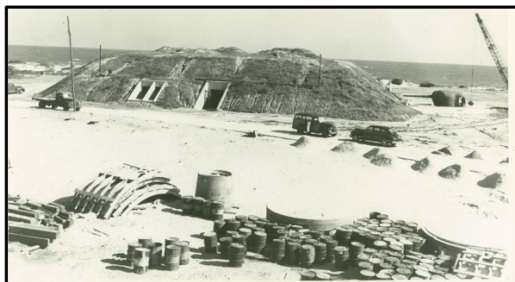
Figure X. Battery Cramer under Construction (Photo housed: NARA)
